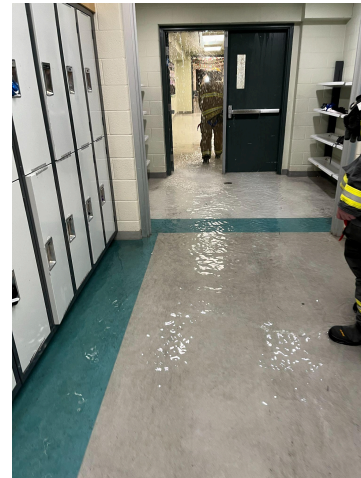
Image of the location of the pipe rupture at FLVT and the water that pooled in on the early morning of Friday, January 12.
